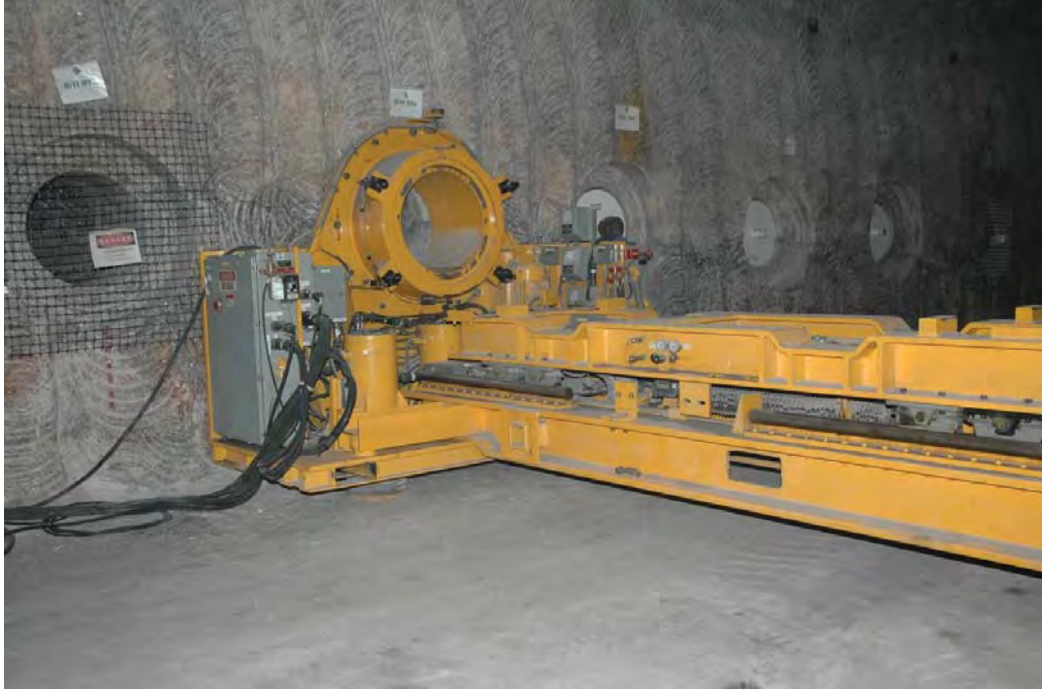
Figure 6 Equipment prepared for RH waste emplacement in Room 2 of Panel 4
