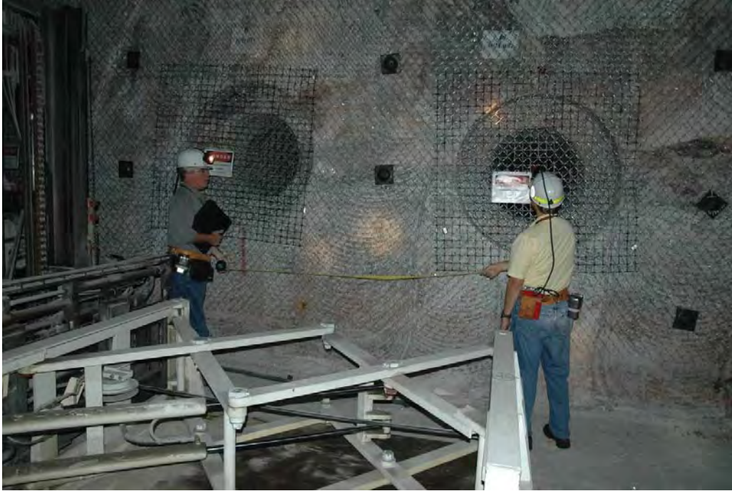
Figure 1 Inspectors check pillar spacing of RH boreholes
